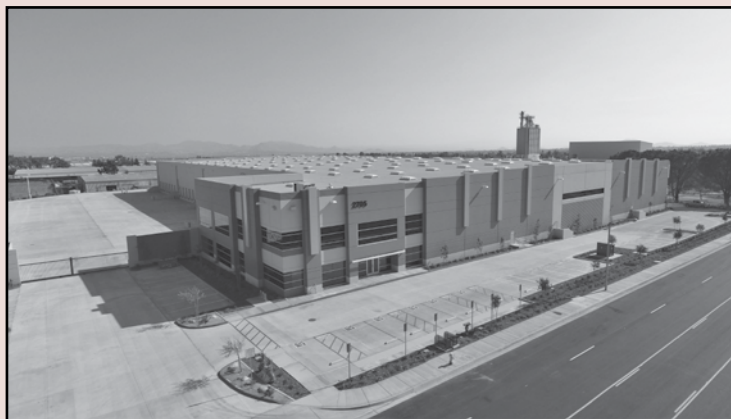
A recently completed industrial asset (warehouse) in California’s Inland Empire region.
